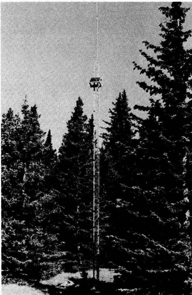
Redondo Peak repeater installation. Solar array is mounted near the top of the tower to prevent shading. The repeater electronics are installed underground at the base of the tower.
