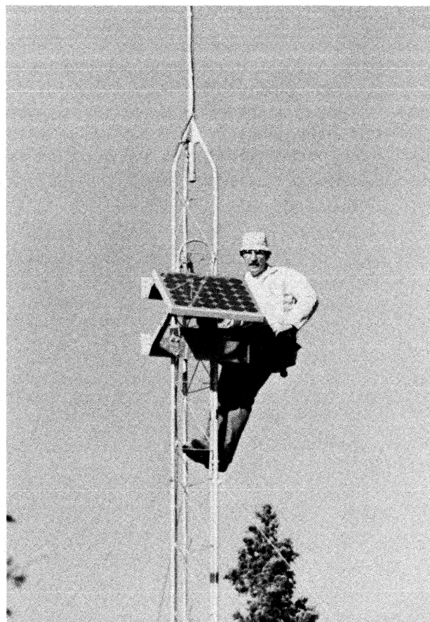
Co-author WB5RSN makes final angle adjustments to solar array that powers the 19-79 repeater on Redondo Peak, New Mexico (3433 meters, 11,254 feet). The array is mounted at 17 meters (55 feet) to prevent shading from nearby trees.
